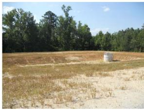
**Photo #8** A dry detention pond was observed in the northern portion of the site.
