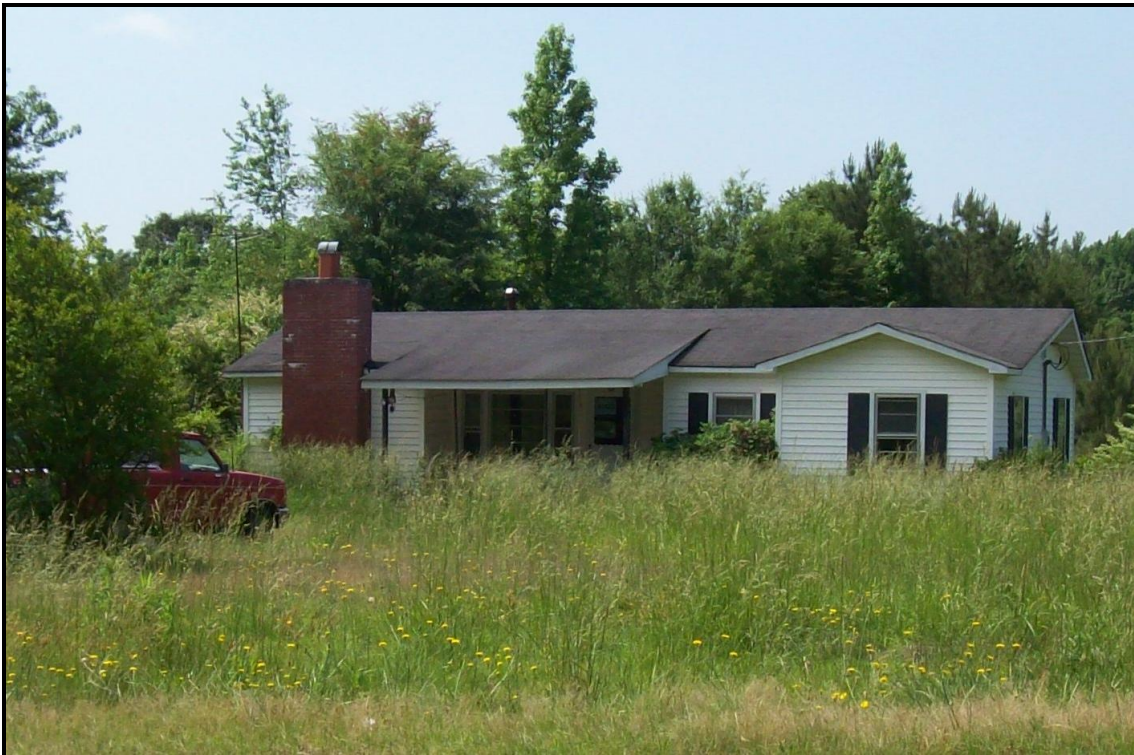
Figure 16. View facing south of Structure 2
