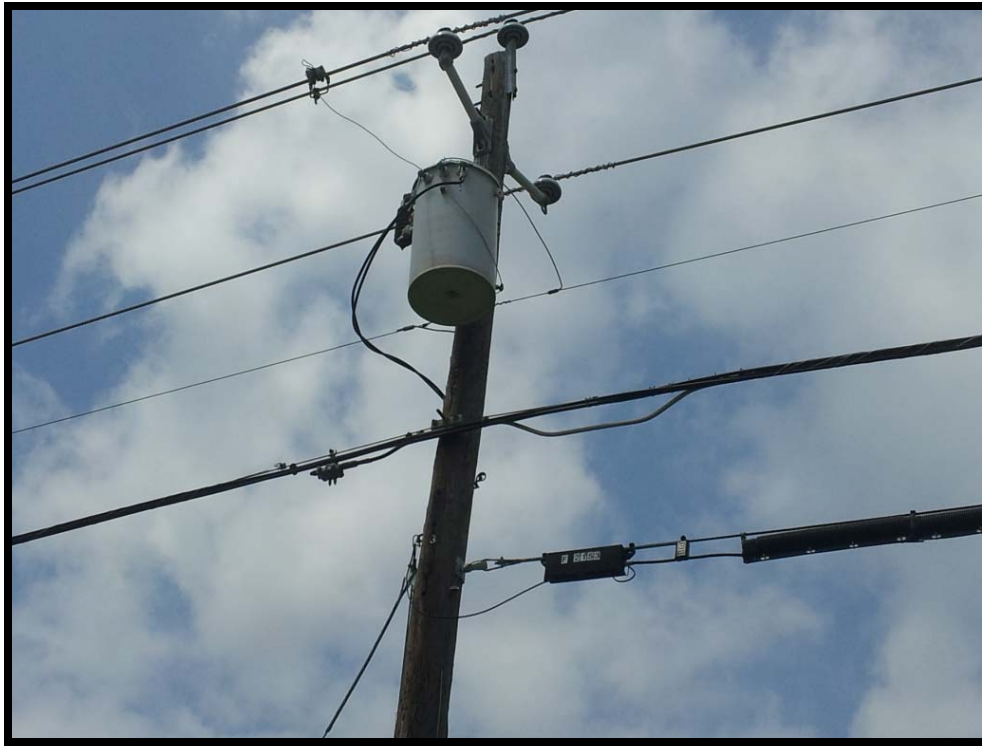
Photograph 5 – Pole mounted transformer located near the property (not leaking)
