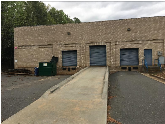
Dock High, Ramp, & Delivery Truck Loading
