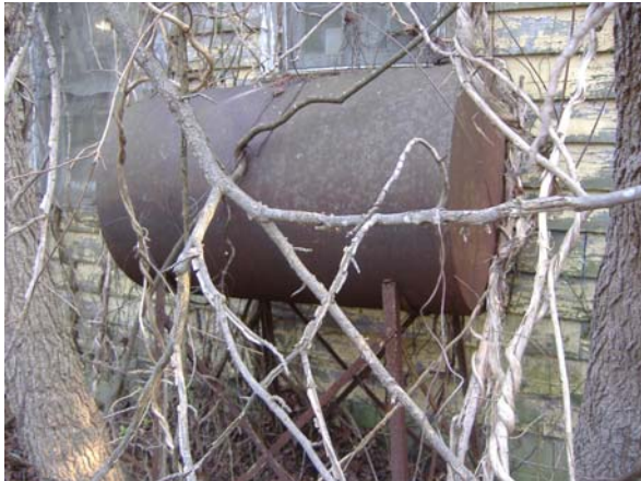
Photo #25 Empty heating oil AST adjacent to dilapidated residence on Tract 3.
