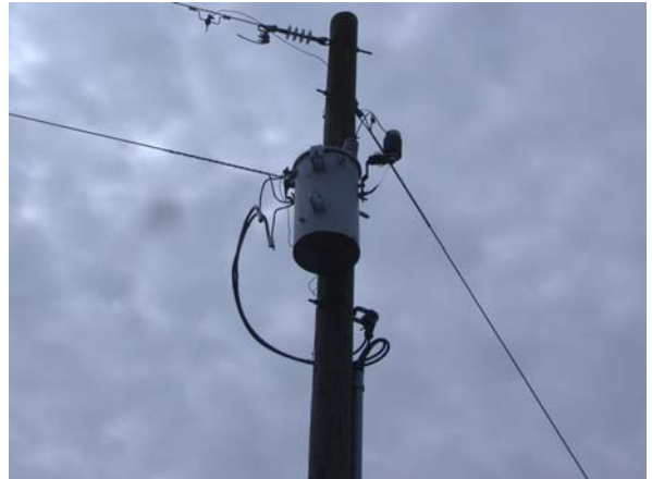
Photo #26 Pole-mounted transformer on Tract 4.
