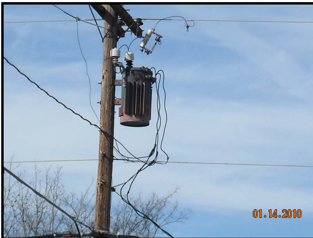
Photograph 38 – Old transformer on northern edge of Lancaster Street (not leaking)
