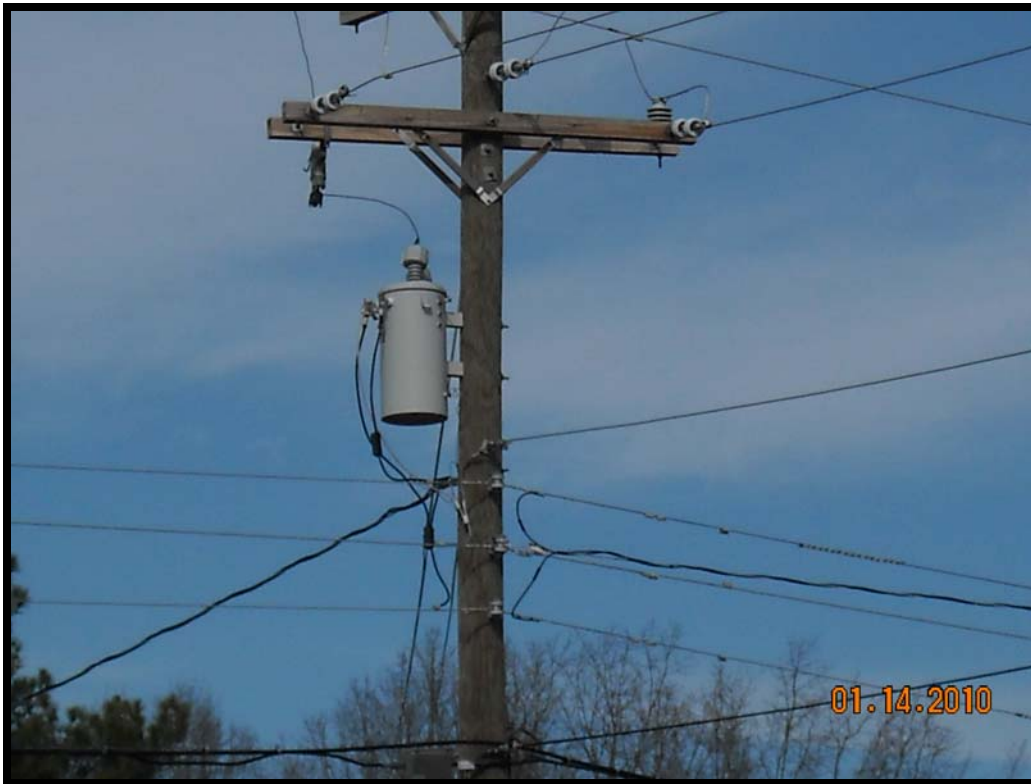
Photograph 33 – Mounted transformer on northern edge of Lancaster Street (not leaking)
