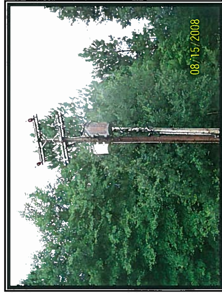
Photo #27 Pole - Mounted Transformer on CCTC Site
